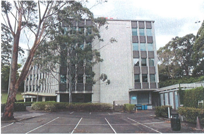
Figure 3.6 3M Building, Pymble South elevation
