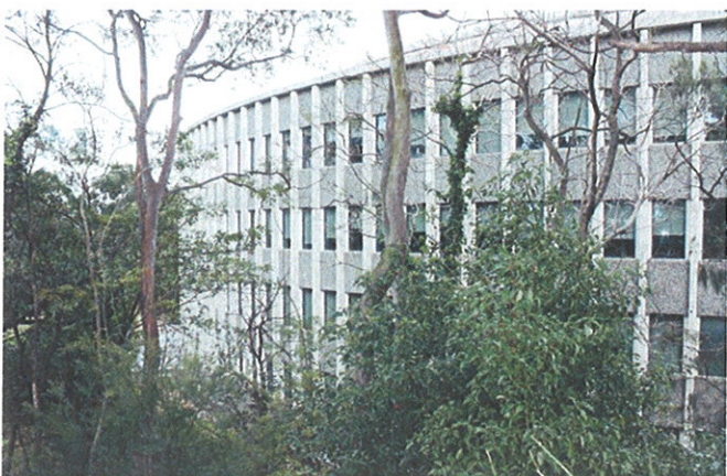
Figure 3.4 3M Building, Pymble Rear elevation
