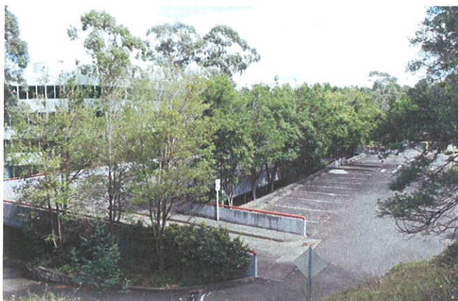
Figure 3.17 3M Building, Pymble Site view looking west
