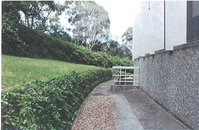
Figure 3.9 3M Building, Pymble Ground floor detail to the rear elevation
