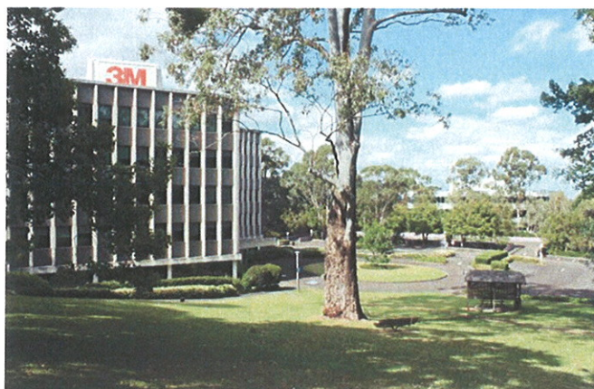
Figure 3.16 3M Building, Pymble Site view looking south east
